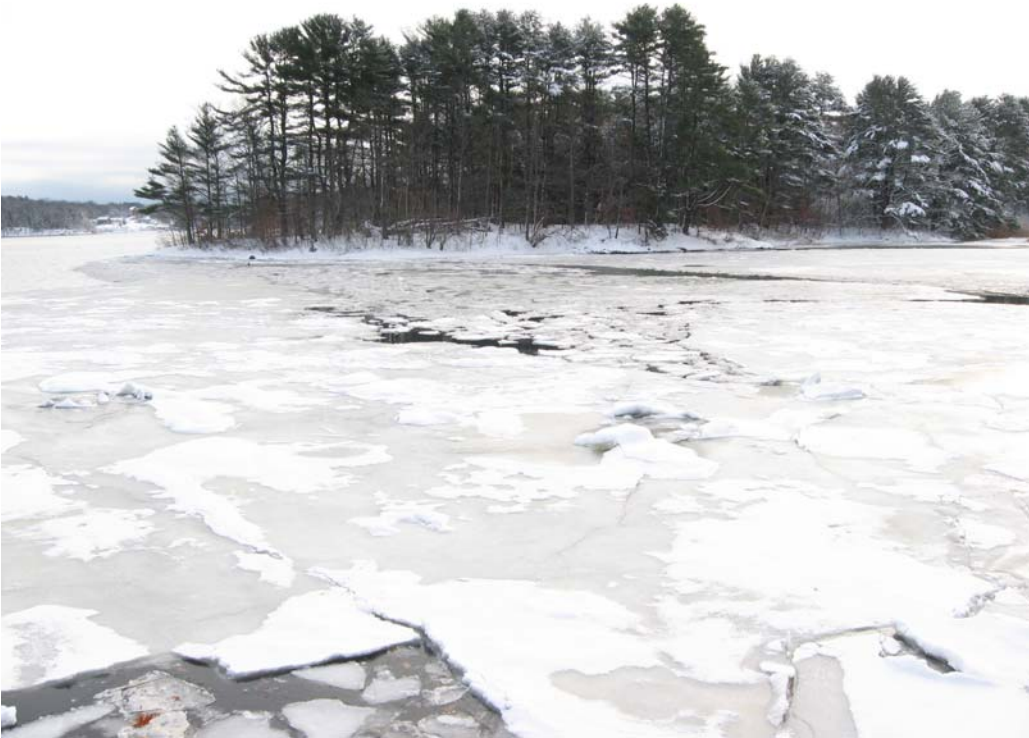
Mill Cove dam near high tide (12/21/07)
